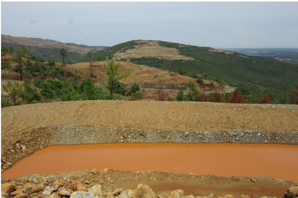
A new nickel slurry tank after the old one was destroyed by a landslide. Photo: Michael Reckordt
